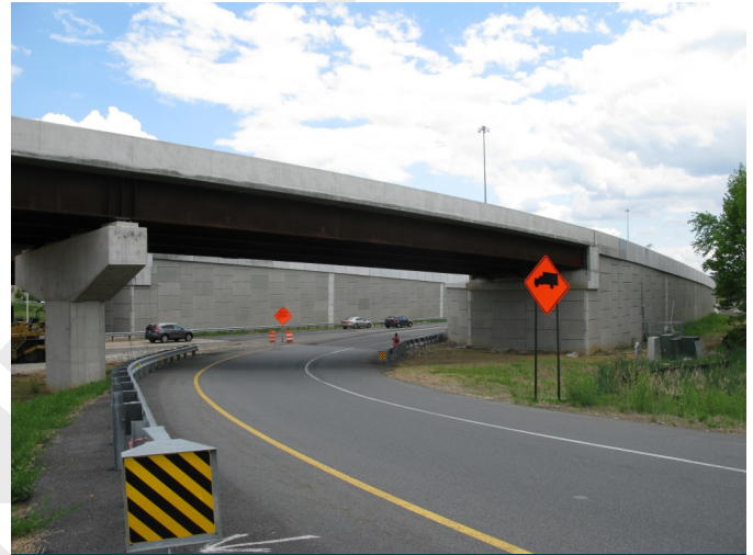
A view of a finished bridge abutment and of a wall
