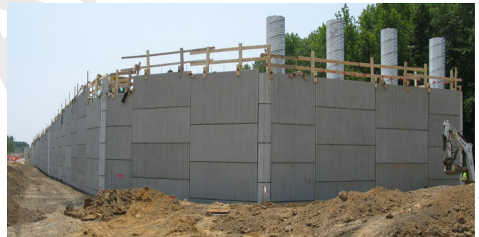
A bridge abutment during - and at the end - of the construction
