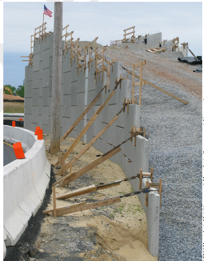
During the construction: the panels and the fill material
