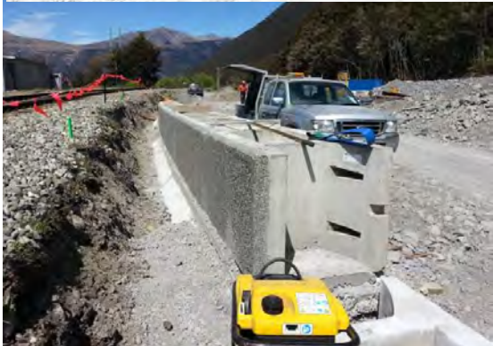
Place initial block on concrete footing, backfill inside block nominal 230mm depth to underside of Paraweb pin connectors with lightly compacted GAP65.
