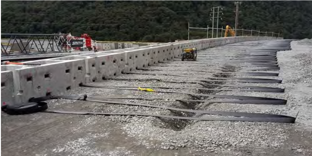
Install nominal 500mm wide, 100mm deep trench 1.5 to 2.0 metres in from rear of MSE block (above). Compact hardfill over rear of Paraweb prior to backfilling and compacting over trench (below).
