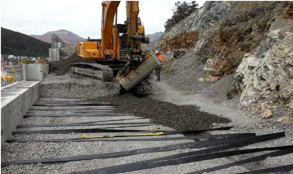
Install nominal 500mm wide, 100mm deep trench 1.5 to 2.0 metres in from rear of MSE block (above). Compact hardfill over rear of Paraweb prior to backfilling and compacting over trench (below).
