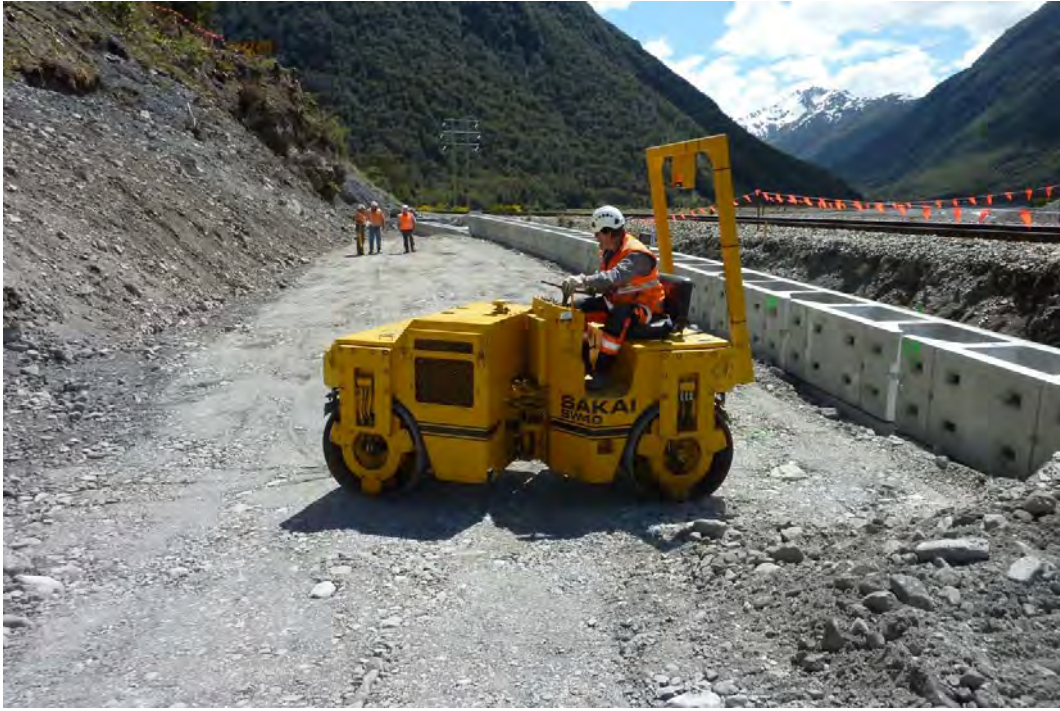
Proof roll MSE reinforced block base (above)
