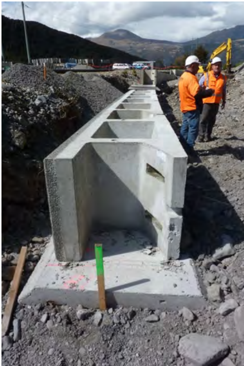
Place initial block on concrete footing, backfill inside block nominal 230mm depth to underside of Paraweb pin connectors with lightly compacted GAP65.
