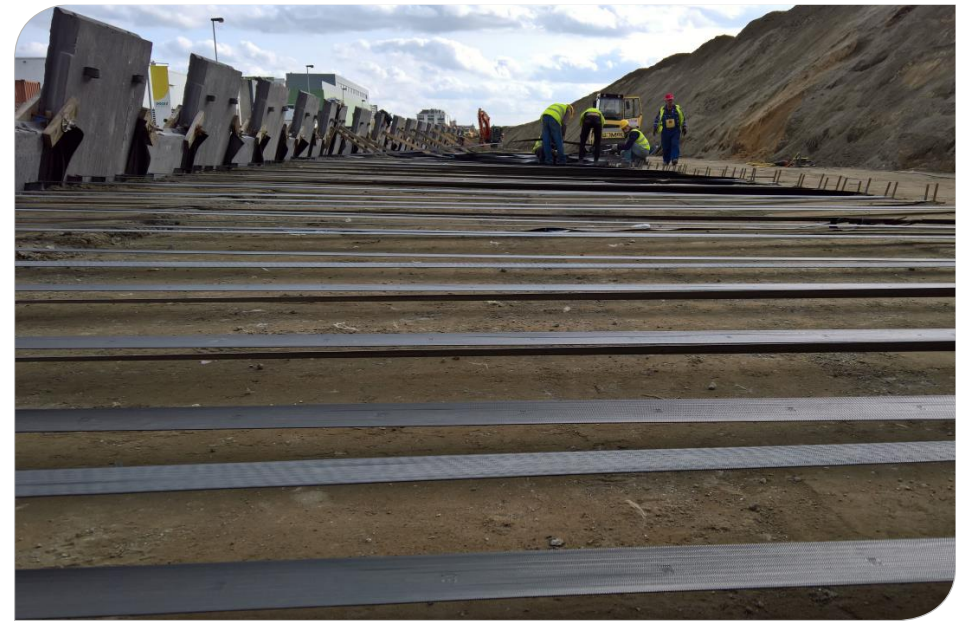
Paraweb used for soil reinforcement
