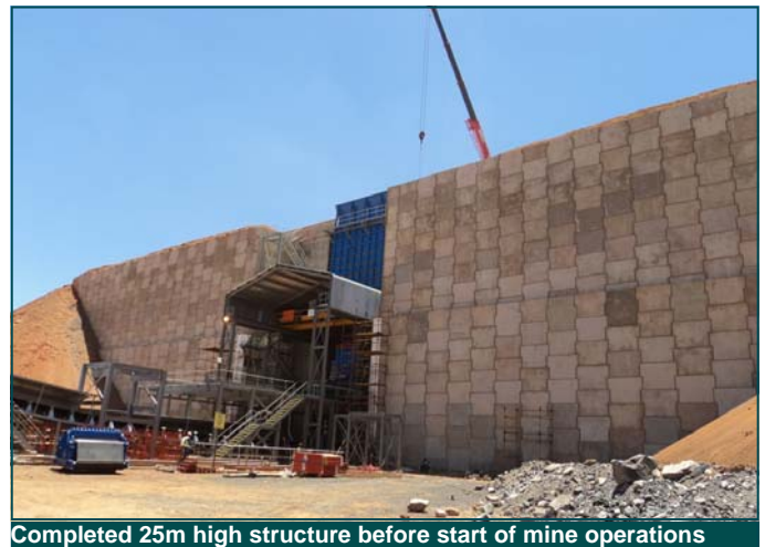
Completed 25m high structure before start of mine operations
