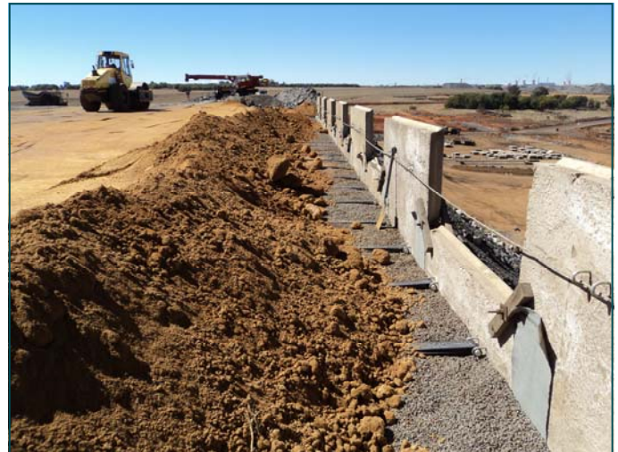
Backfilling and compaction in MacForce construction
