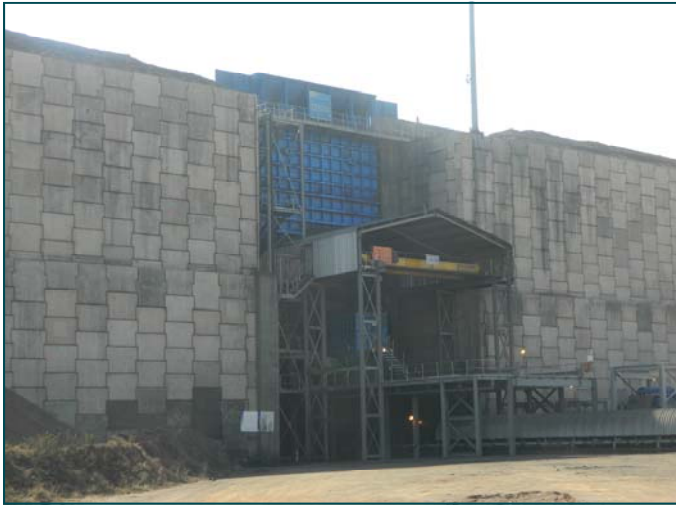
Completed 25m high structure during mine operations
