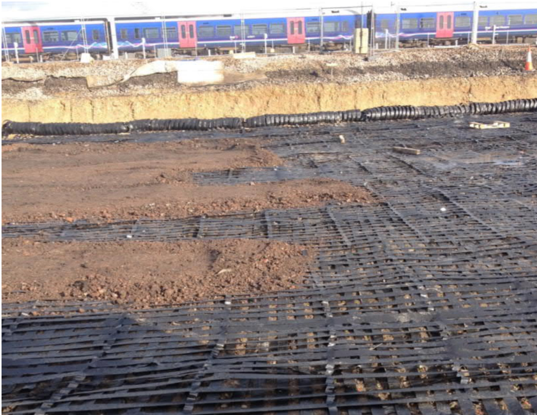
Figure 2 – Load Transfer Platform with ParaLink® - March 2014
