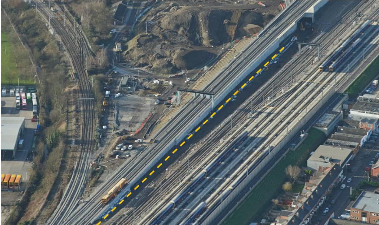
Figure 9 – Aerial View of East Ramp
