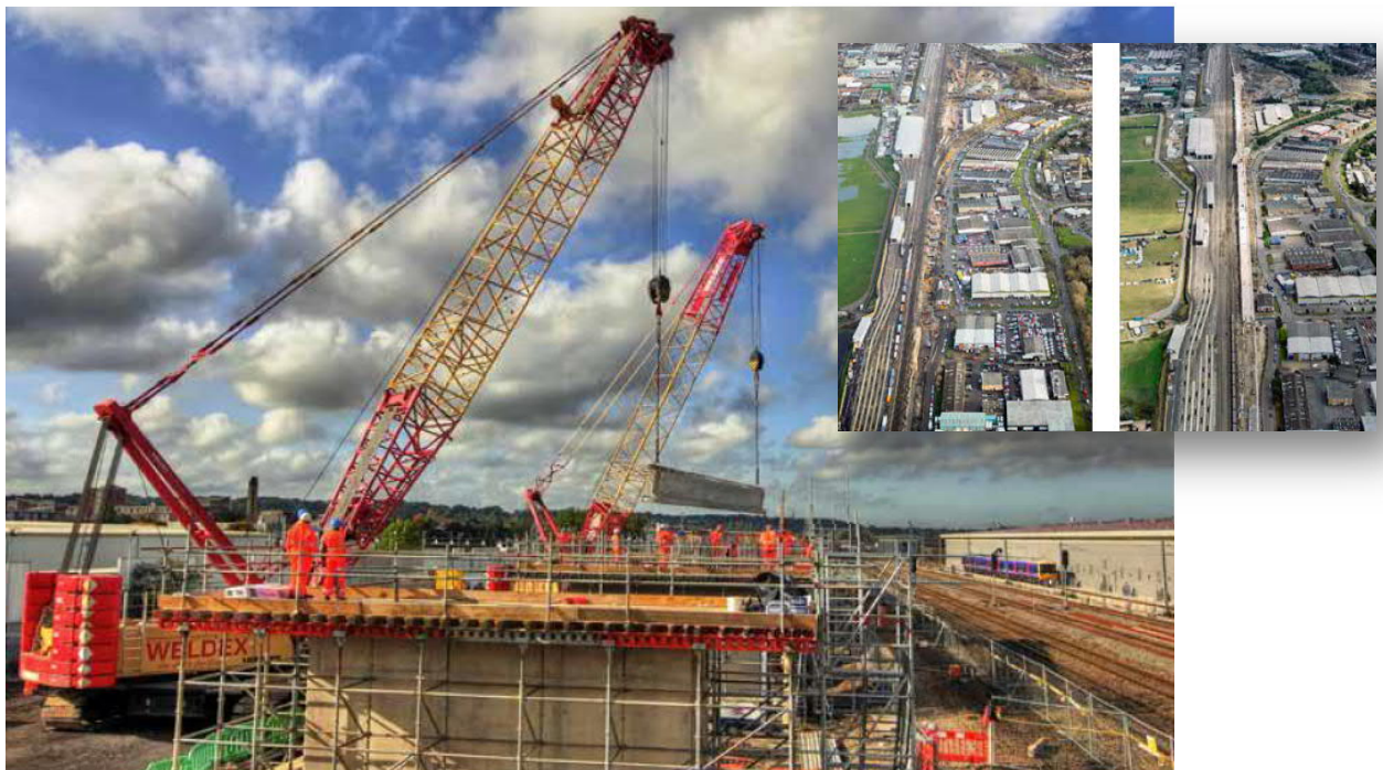
Figure 1 – New Viaduct construction by Balfour Betty
