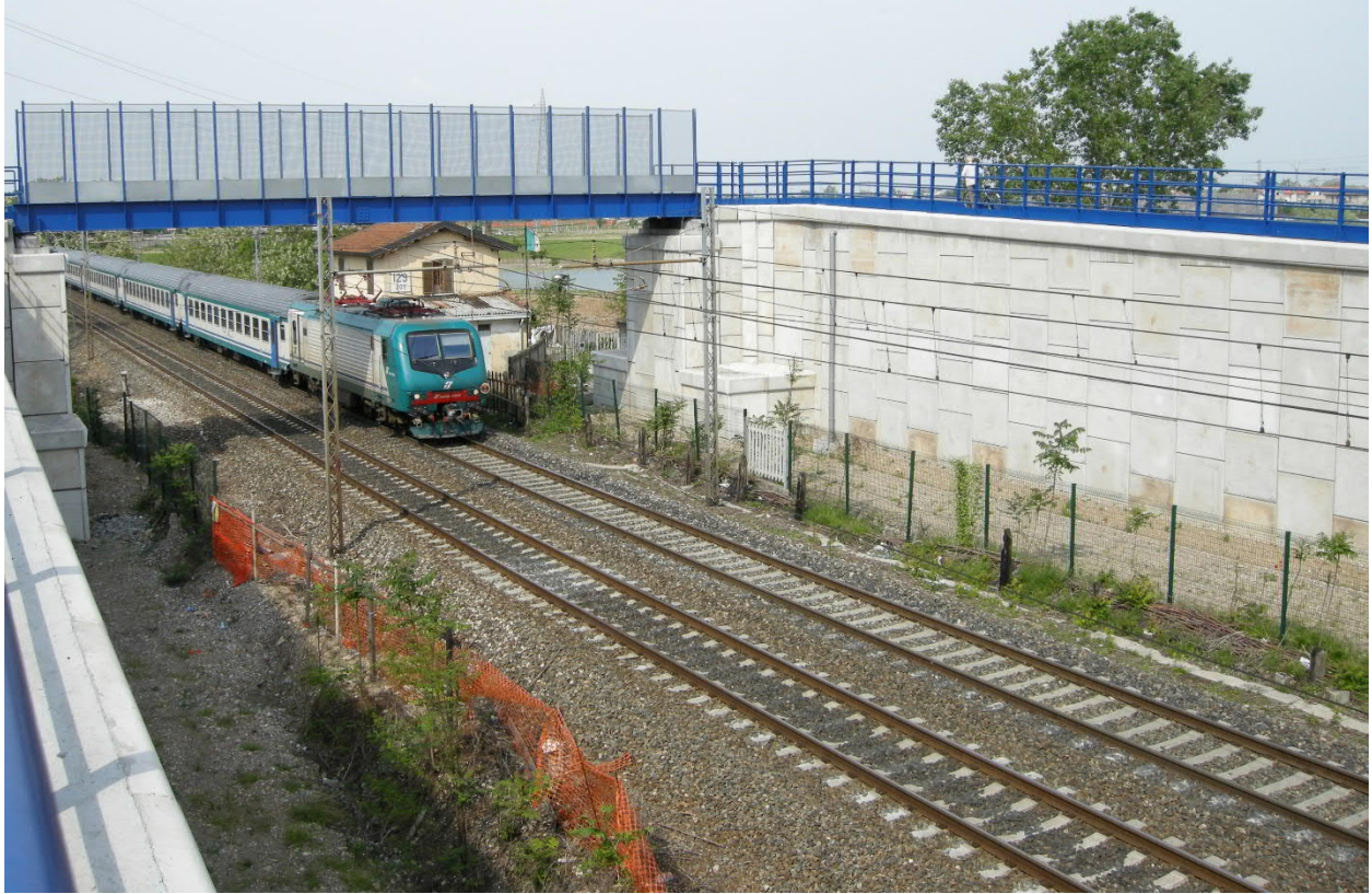
Figure 14 – End of Construction (July 2008)
