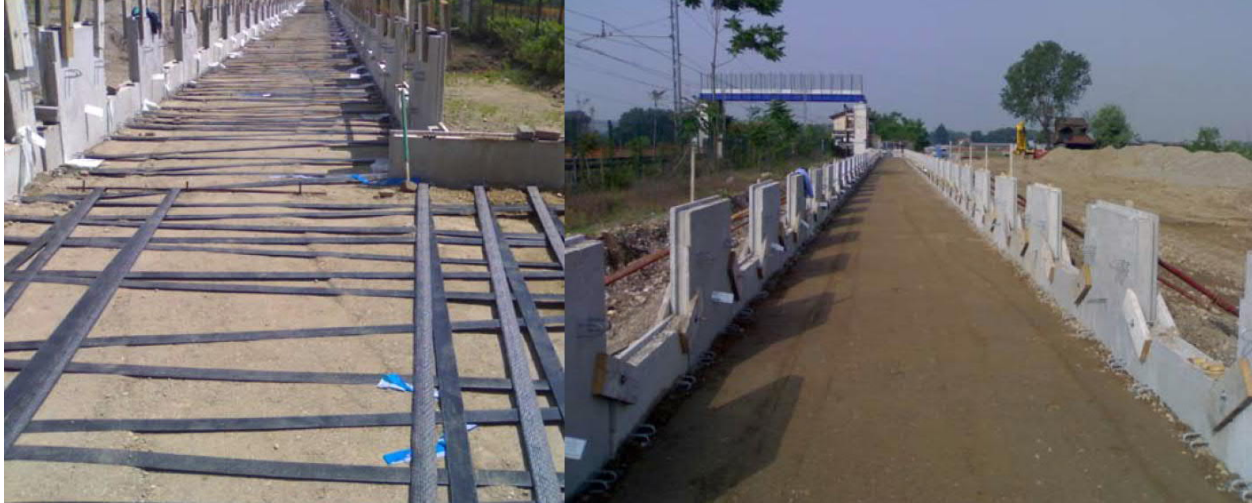
Figure 12 - MacRes® System Installation
