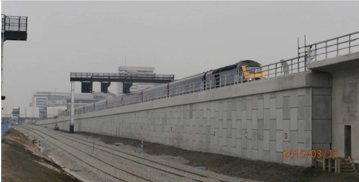
Figure 7 – Reading viaduct MacRes® structure
