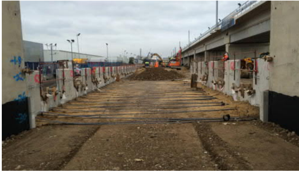
Figure 5 – Festival Ramp Under Construction (November 2014)
