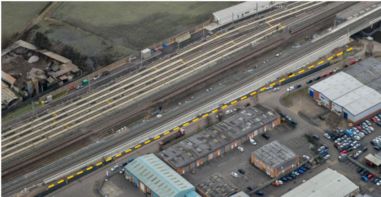
Figure 8 – Aerial view of West Ramp
