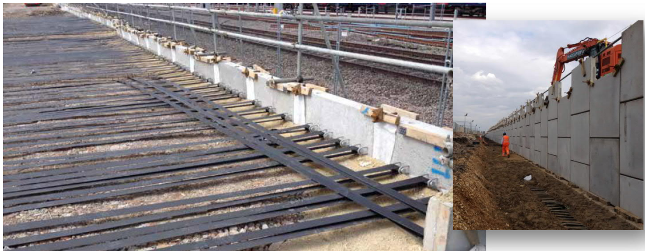
Figure 4 - West Ramp During Construction
