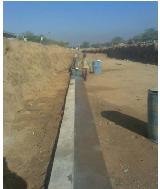
Photo 1. Construction of leveling pad
