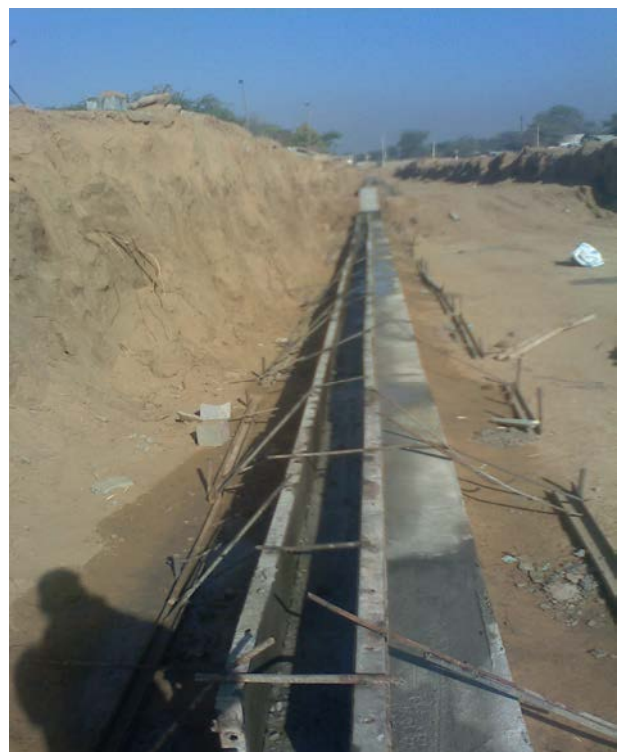
Photo 2. Initial Stage of panel erection
