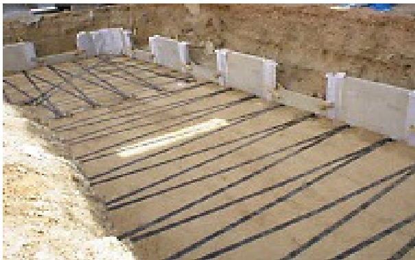
Photo.3,4 Erection & Laying of Facia Panel
