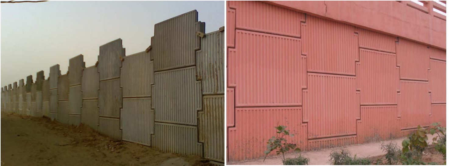
Photo. 6,7 Completion of Panel Erection
