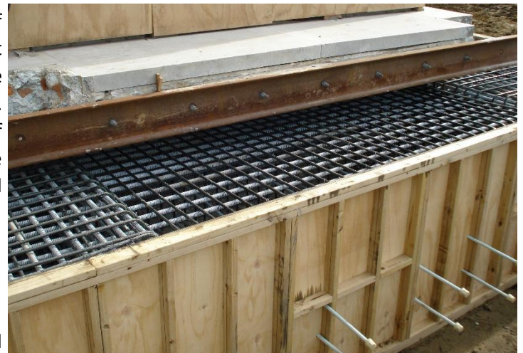
mateenbar™ ring foundation in situ, with formwork held by mateenbolt
