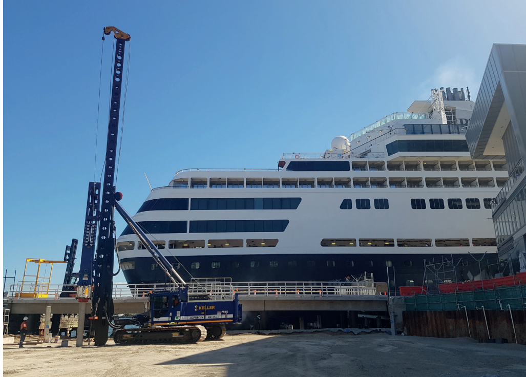
Fig.2: Completed working platform
