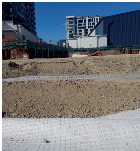
Fig.3: Combigrid® and Secugrid® reinforced working platform
