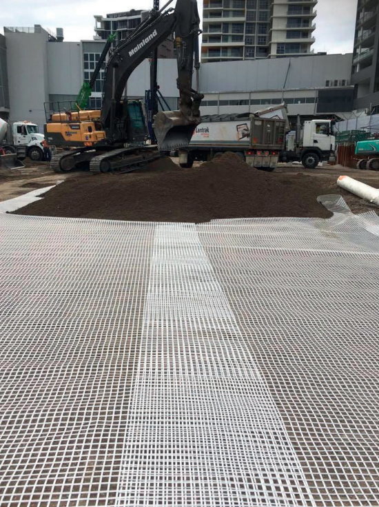
Fig.1: Covering Secugrid® with subbase material
