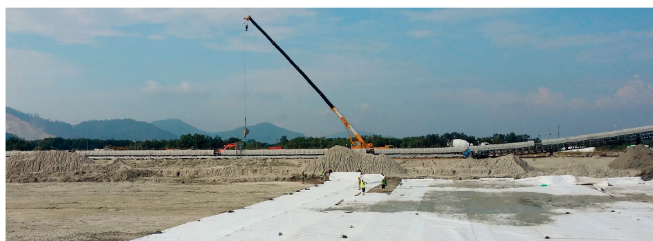
Fig.2: Water from saturated soft marine clay reflected on Combigrid® layer
