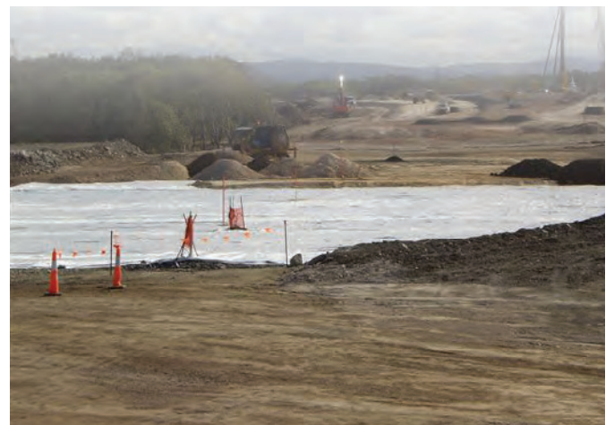
ACETex® PET structural geotextile Northern Access Road Project Brisbane, QLD
