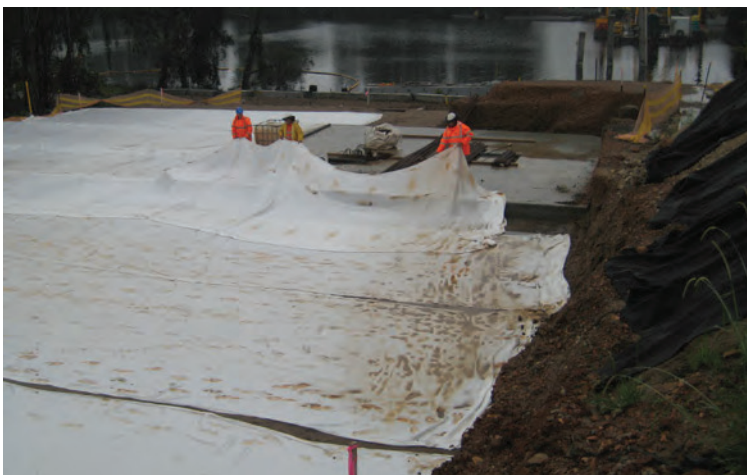
ACETex® PET structural geotextile Coopernook Bypass Project Coopernook, NSW
