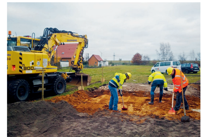
Figure 5: Uncovering of Secugrid® HS to determine the installation damage ( RF_{CR} ) reduction factor
