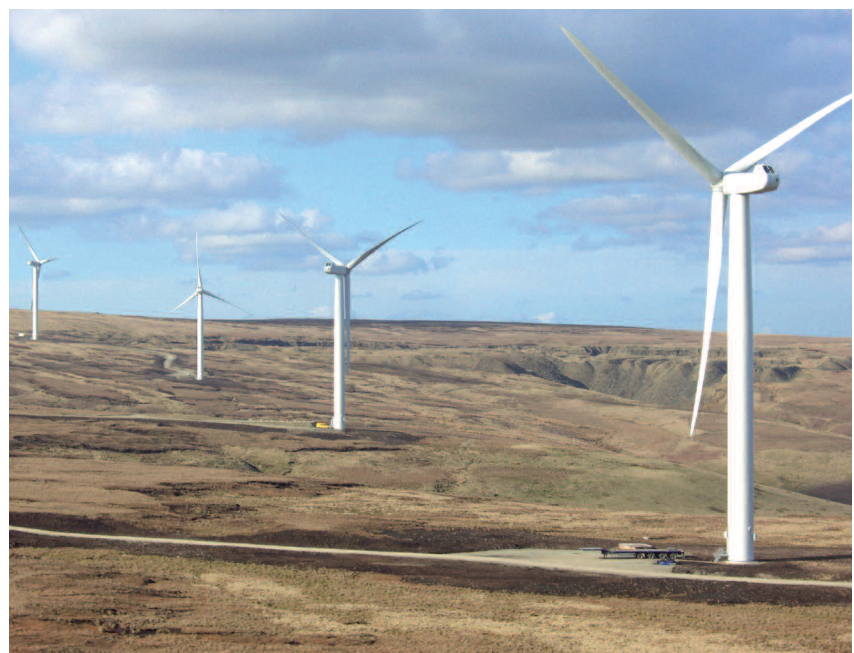
Figure 4 Finalised windfarm with Secugrid® soil reinforced areas
