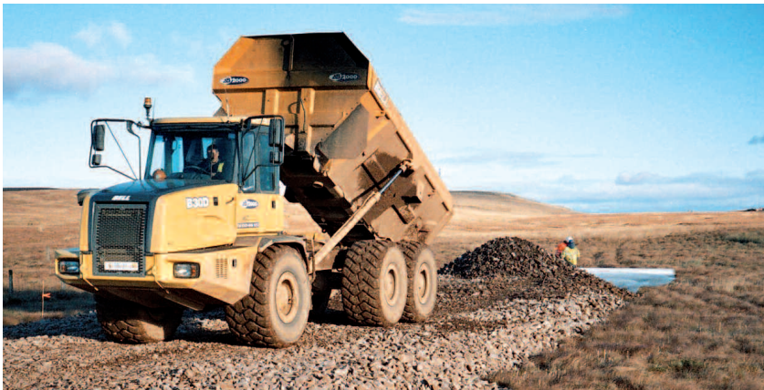
Figure 3 Placement of aggregate on Secugrid®
