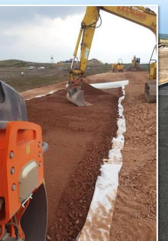
For the hardstanding area, Craddys' design specification utilised three separate layers of Secutex® Green 30G1 GRK 2...
