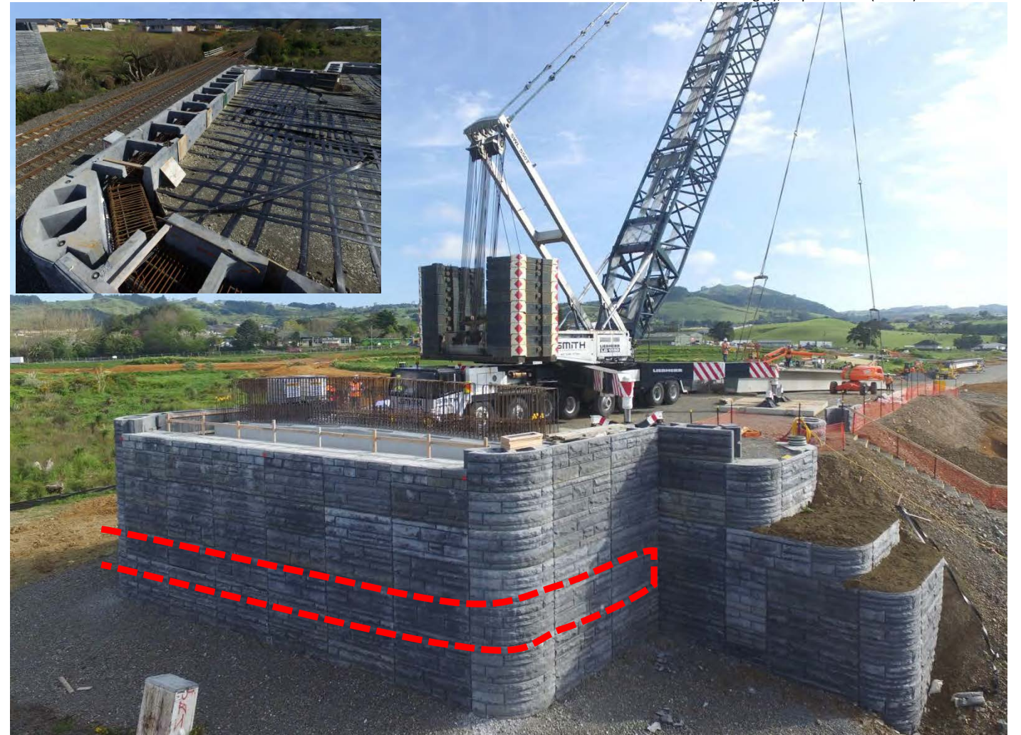
Circular corner blocks (above right); Impact beam (below)
