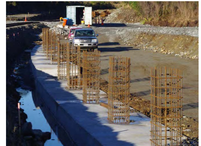
Paraweb & block fittings (top) abutment foundation (above), looking south between both abutment walls (below)
