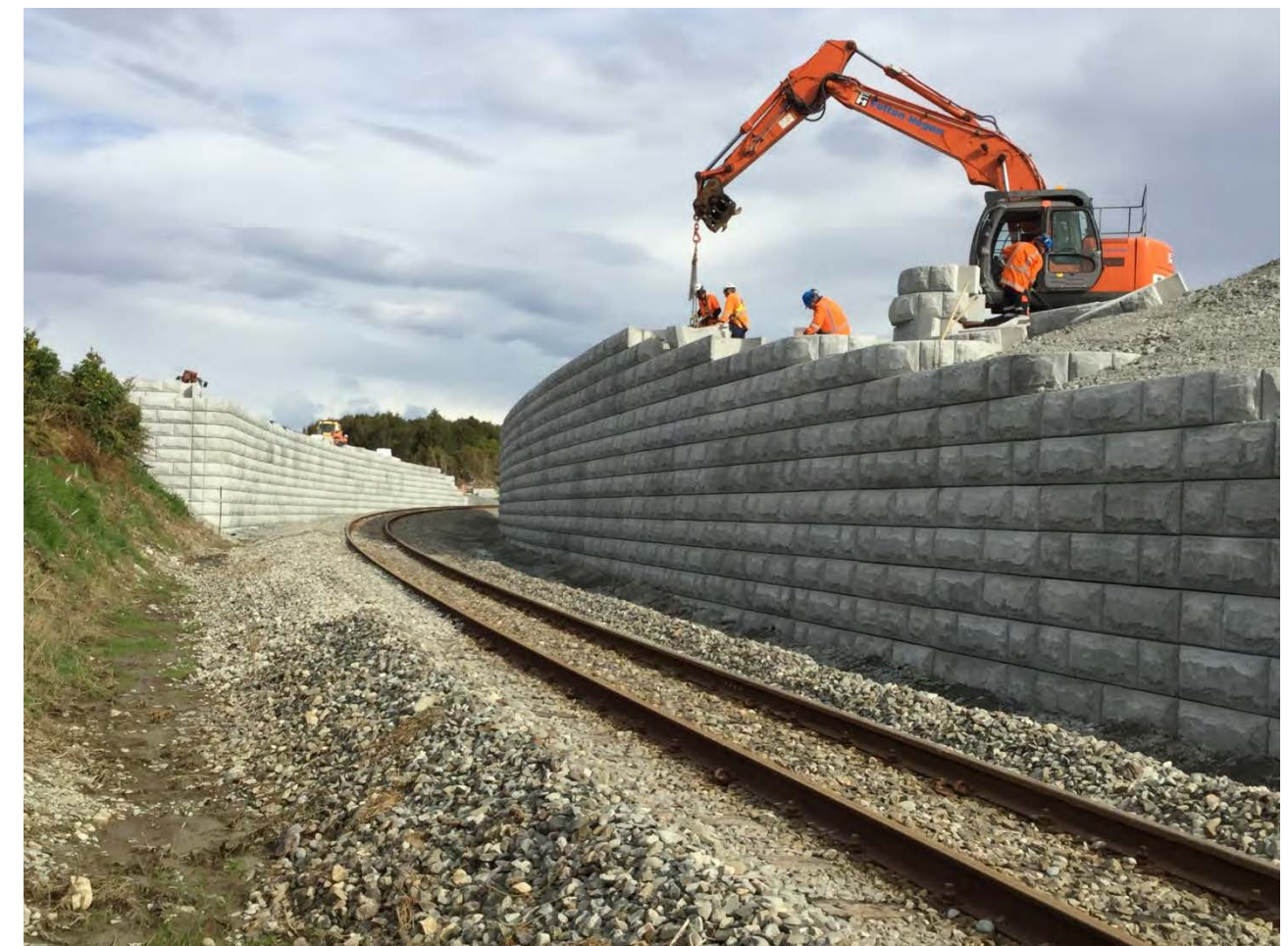
Paraweb & block fittings (top) abutment foundation (above), looking south between both abutment walls (below)
