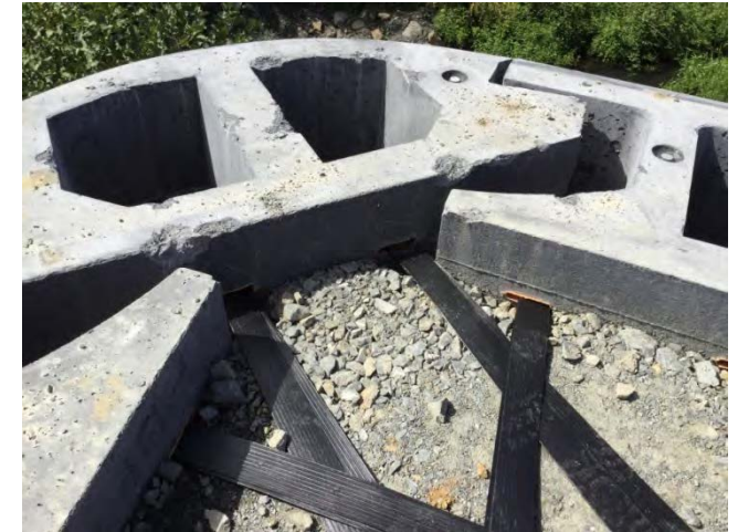
Circular corner blocks (above right); Impact beam (below)
