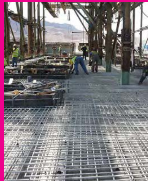
Potash Plant Concrete Slab Replacement, Jordan
