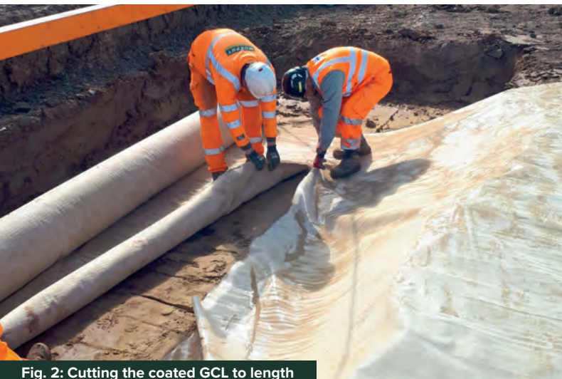
Fig. 2: Cutting the coated GCL to length
