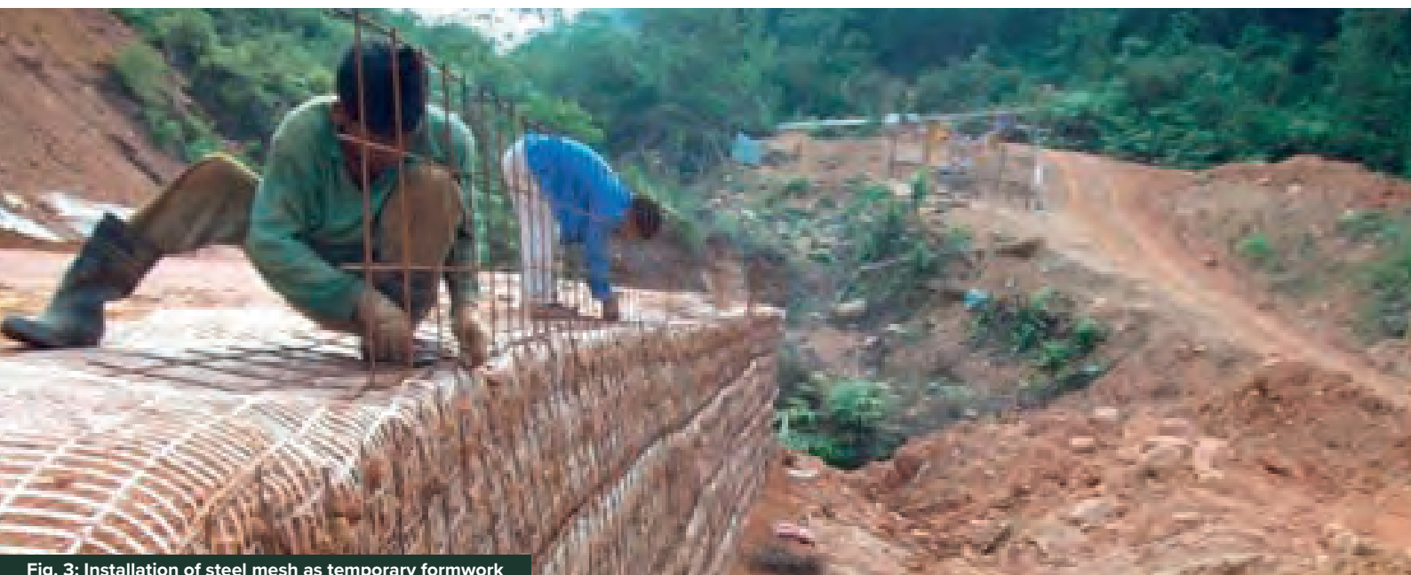
Fig. 3: Installation of steel mesh as temporary formwork
