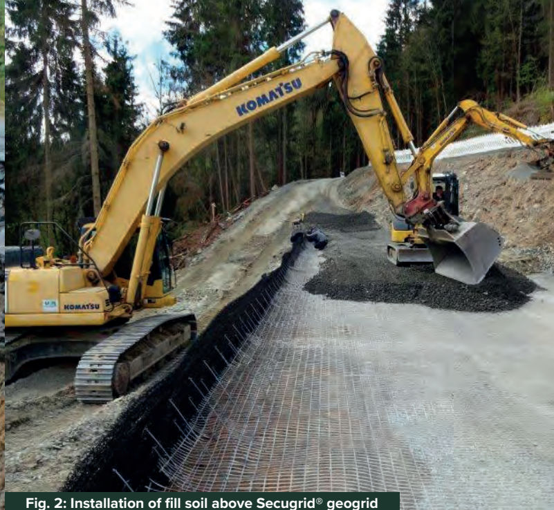
Fig. 2: Installation of fill soil above Secugrid® geogrid
