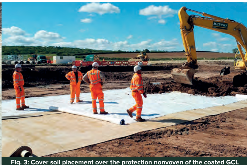
Fig. 3: Cover soil placement over the protection nonwoven of the coated GCL
