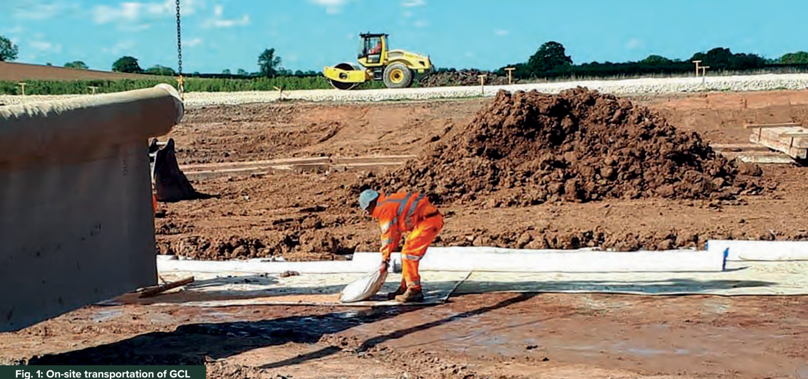
Fig. 1: On-site transportation of GCL
