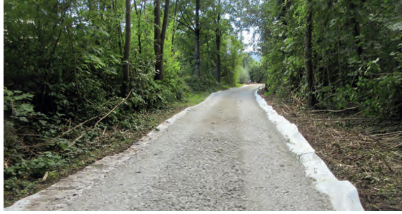
Fig. 2: Construction road on the island between mill canal and Lauter
