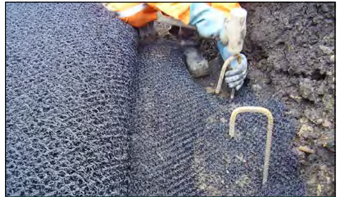
Fixing MacMat in trench
