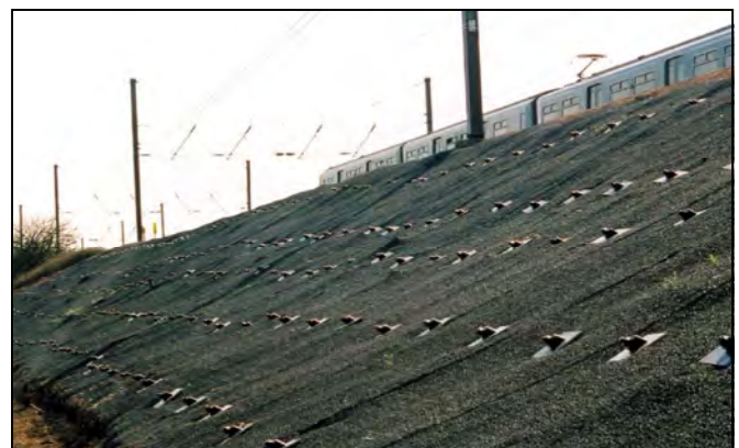
MacMat® R and soil nail reinforced slope
