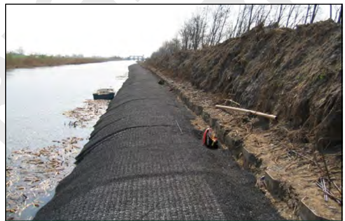
MacMat® R erosion protection on river bank
