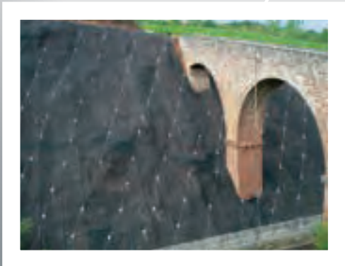
Soil nailing and Surface protection
