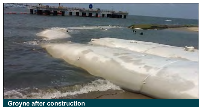
After construction of 500 m long protection bund structure
