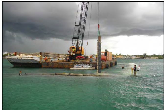
Maccaferri Polymeric Marine Mattress installation
