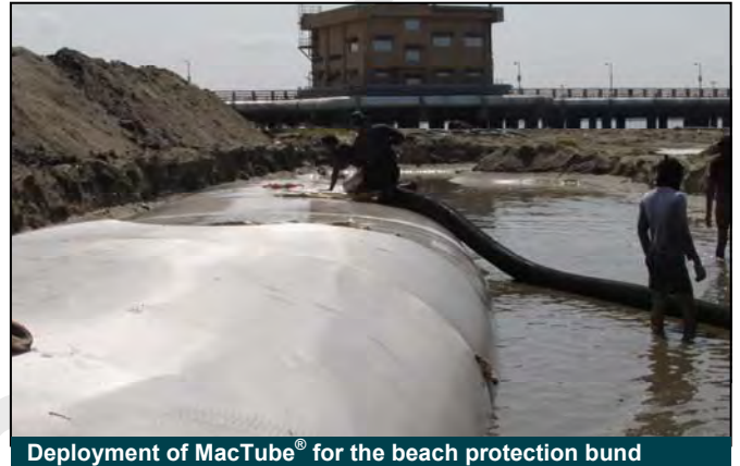
Deployment of MacTube® for the beach protection bund
