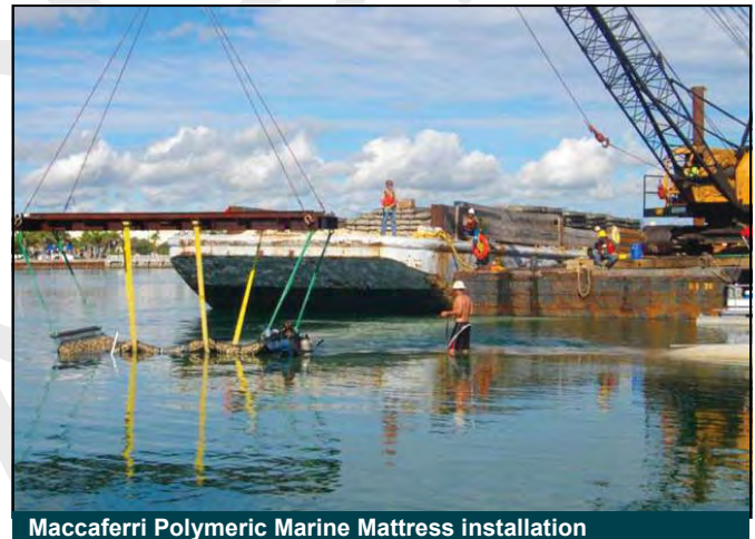
Maccaferri Polymeric Marine Mattress installation
