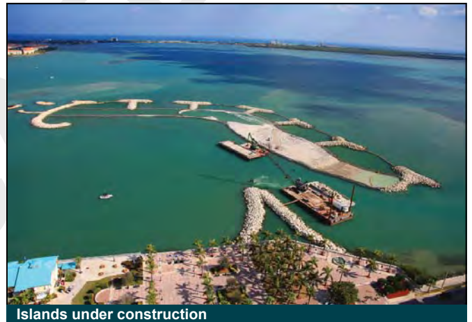
Islands under construction
