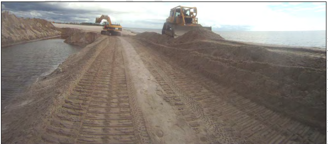
Final beach fill coverage over MacTube® / MacScour, to surface level
