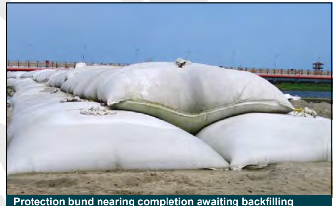
Protection bund nearing completion awaiting backfilling
