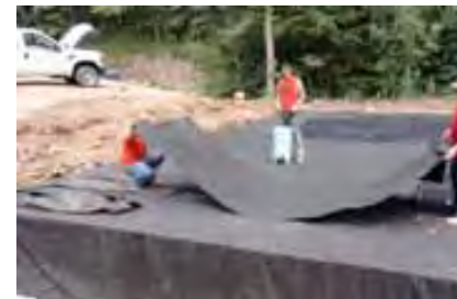
Fig. 20 Encapsulate Ellipse Tanks with
