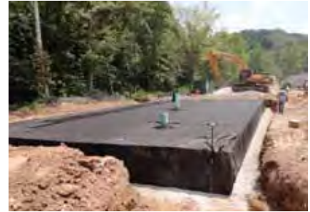
Fig. 22 “Walk” the geotextile into the corner to eliminate folds & air gaps.
