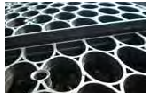
Fig 9A: Minor variations (less than width of the top plate) in height are acceptable.
