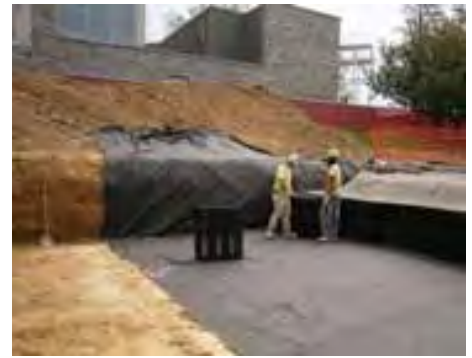
Fig 6: Pull Wrinkles out of Geotextile so Material lays flat.
