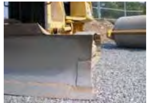
Fig. 5 Base must be smooth to ensure units fit together without gaps.
