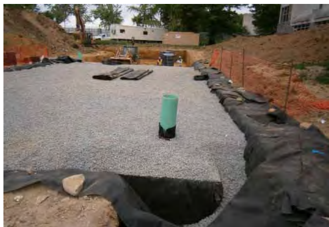
Fig. 24 Use an LGP dozer to push backfill over Ellipse Tank units.
