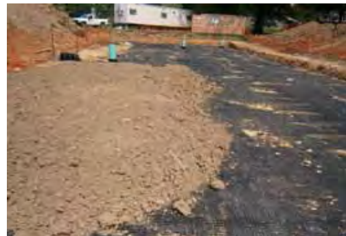
Fig. 25 Overlap Geogrid 300mm or as required by plans.
