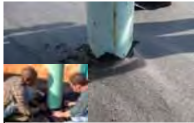
Fig. 19 Cut an “X” into textile to accommodate pipe penetration.
