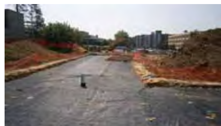
Fig. 25 Overlap Geogrid 300mm or as required by plans.
