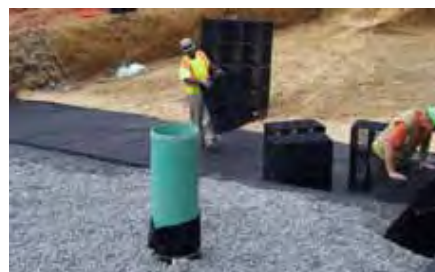
Fig 11: Installed inspection Port
