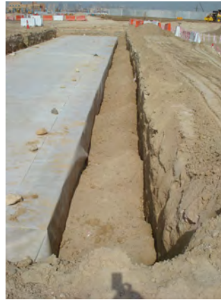
Fig. 23 Vibratory compaction of side backfill is always required , regardless of what backfill material is used.
