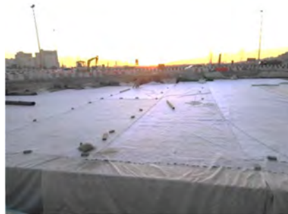
Fig. 13 Maintain 300mm overlap on with geotextile
