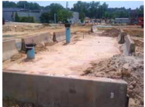
Fig. 21 Secured STORMVAULT Tank installation using Jersey Barriers.
