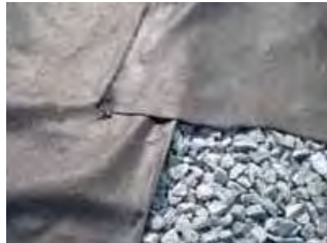
Fig 9: Reduced overlaps don't create significant savings and can create delays.
