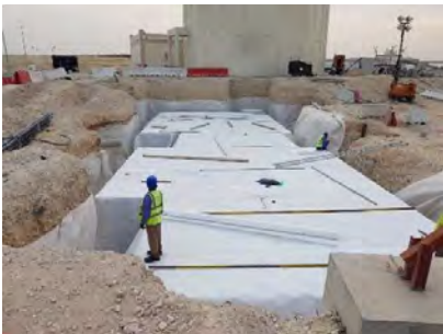
Fig. 12 Encapsulate STORMVAULT Tanks with geotextile
