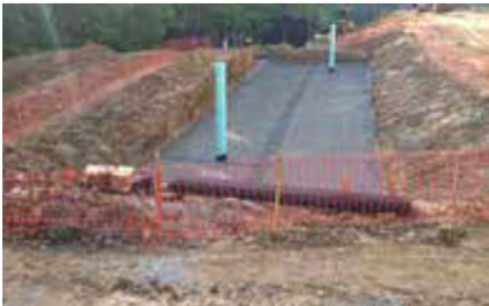
Fig. 20 Secure the installation with temporary fencing.
