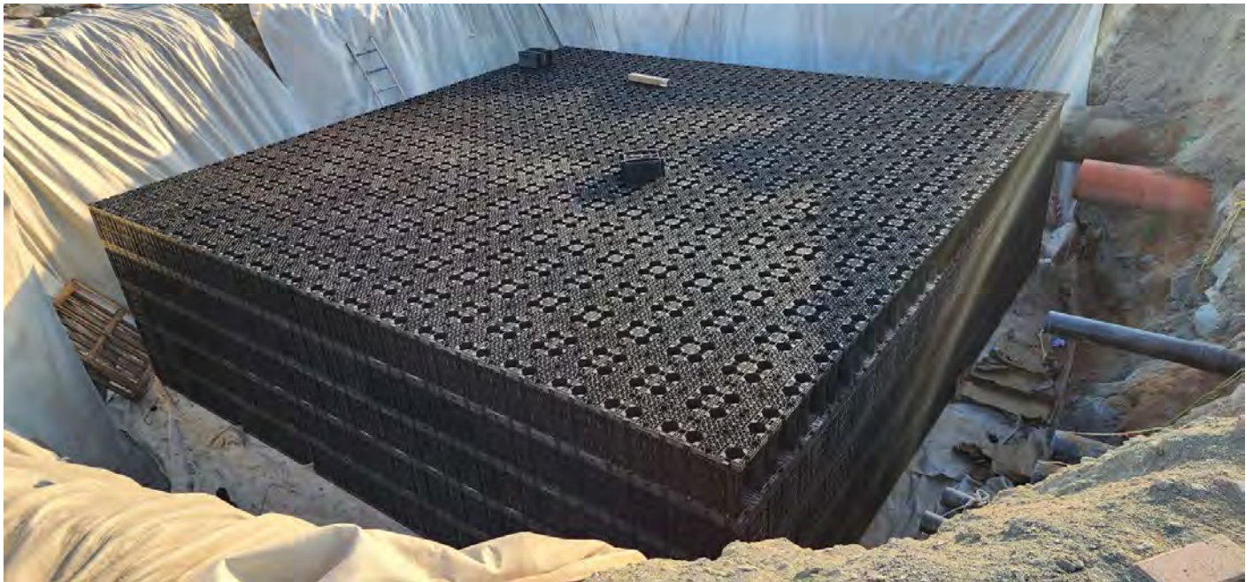
Fig 11: Plan view showing all units installed in a brick laying pattern.
