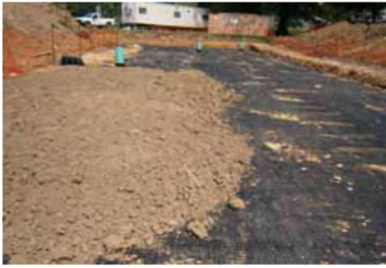
Fig. 19 Pushing backfill parallel to the Geogrid.
