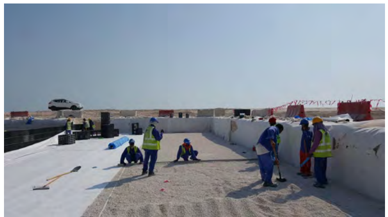
Fig. 3 Compacted and Levelled subbase to 95% proctor
