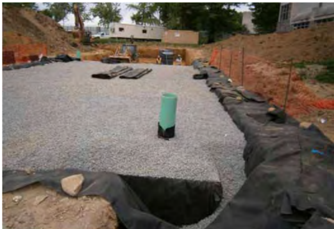
Fig. 17 Use an LGP dozer to push backfill over STORMVAULT Tank units.
