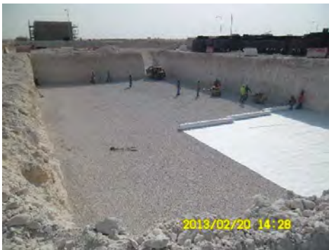
Fig 8: Overlap Geotextile by minimal 300mm or more. Pull Wrinkles out of Geotextile so Material lays flat.
