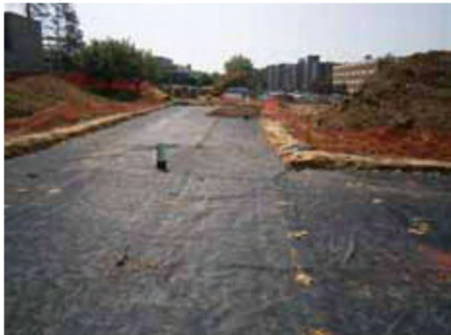
Fig. 18 Overlap Geogrid 300mm or as required by plans.
