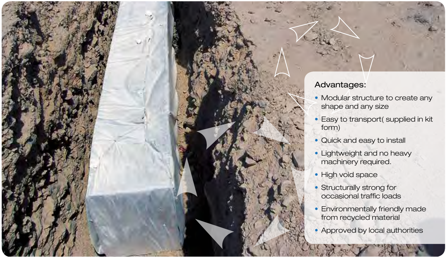
Septic Leach Drain System (side view A-A)
